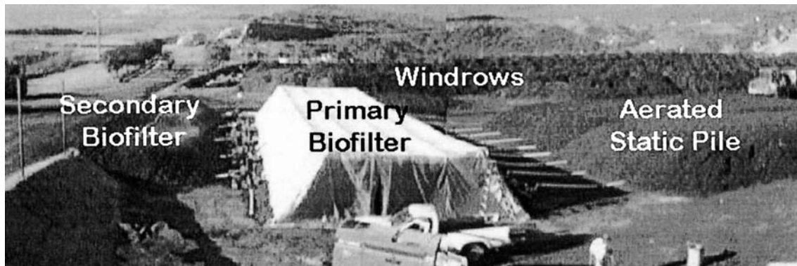
Figure 2—Photo of windrows, aerated static pile, and primary and secondary biofilters.
